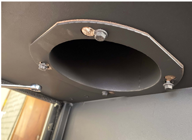
1. Loosen two of the bolts diagonally.
